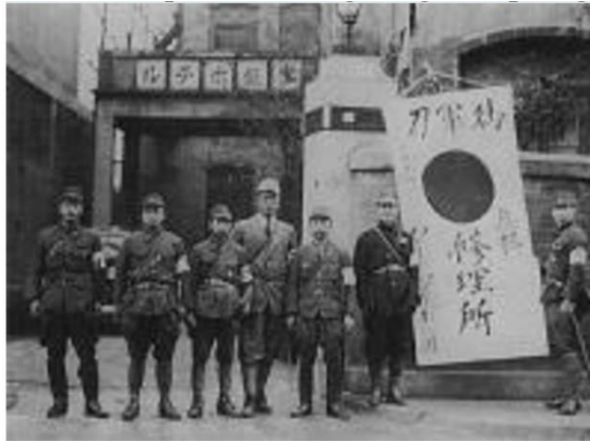
Shigetsugu's repair group in front of the Army Sword Repairing Factory.
